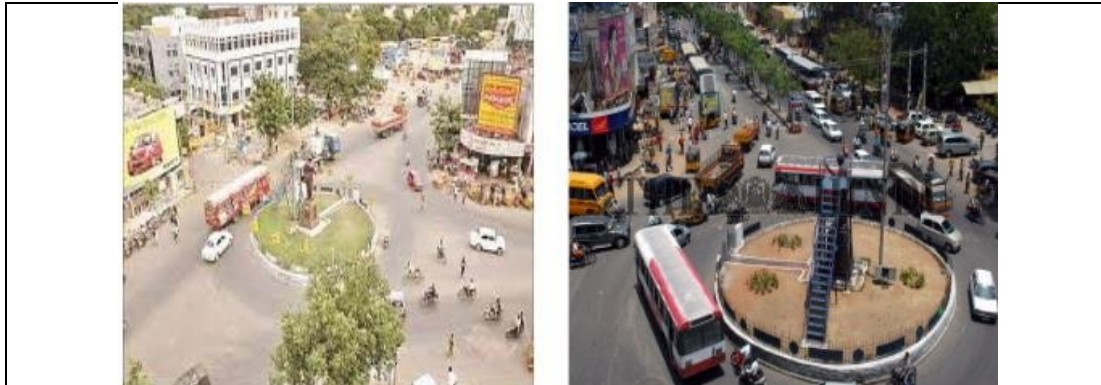
Figure 1: Aerial View of the Study Intersection
